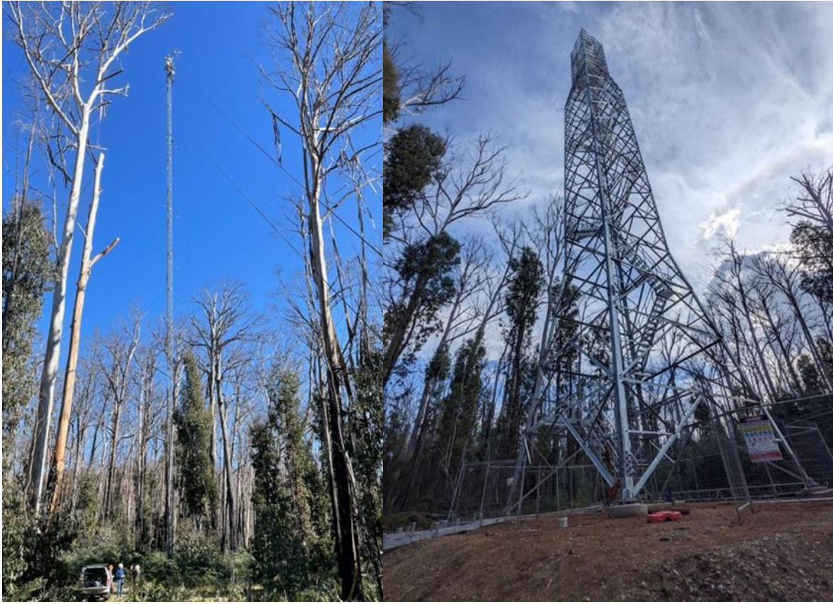
The old Tumbarumba tower after the 2019/20 summer (right). The new tower is nearing completion, it is a free-standing tower with an internal staircase (left).
