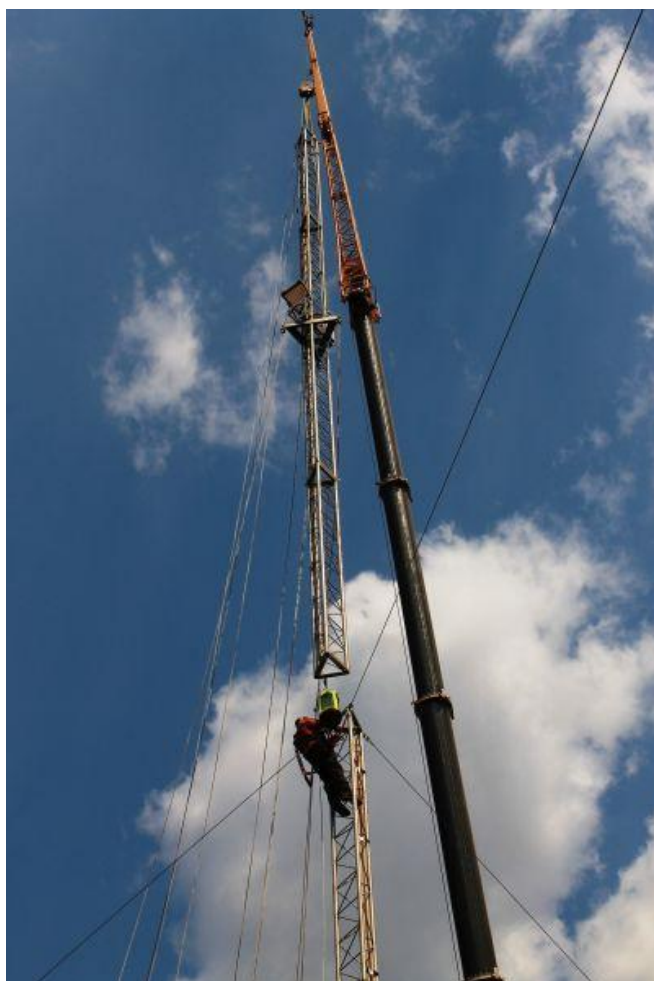
Litchfield flux tower under construction. (Photo by Karen Joyce)
