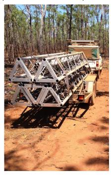
Tower update: The concrete problems have been fixed with a series of rods embedded through the blocks and the tower sections are *en route* to the site for erection
